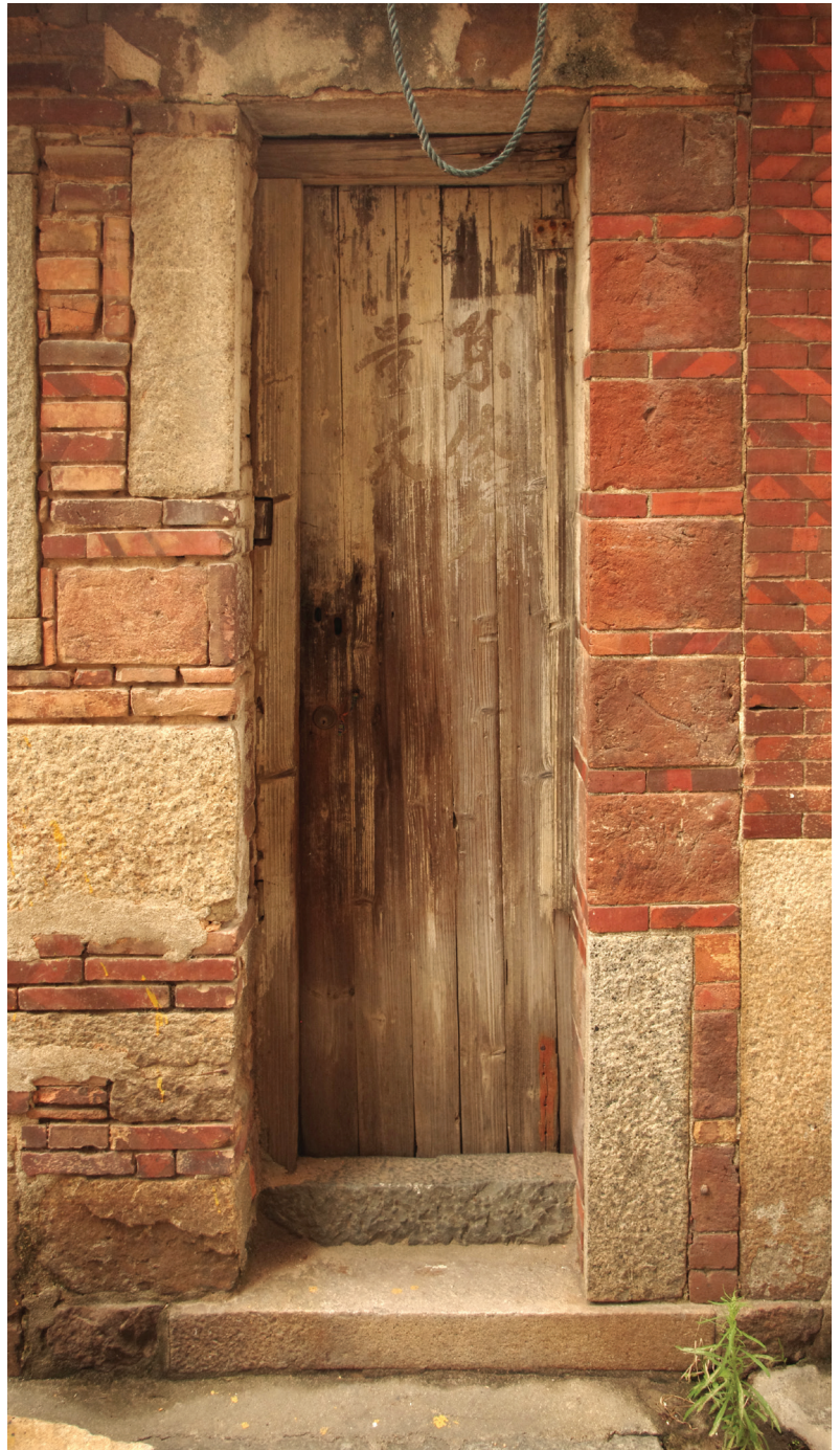
Fig. 6: A narrow side door of a residence in the ancient center of Anhai. The use of facing bricks and large granite slabs characterizes the traditional architecture.
